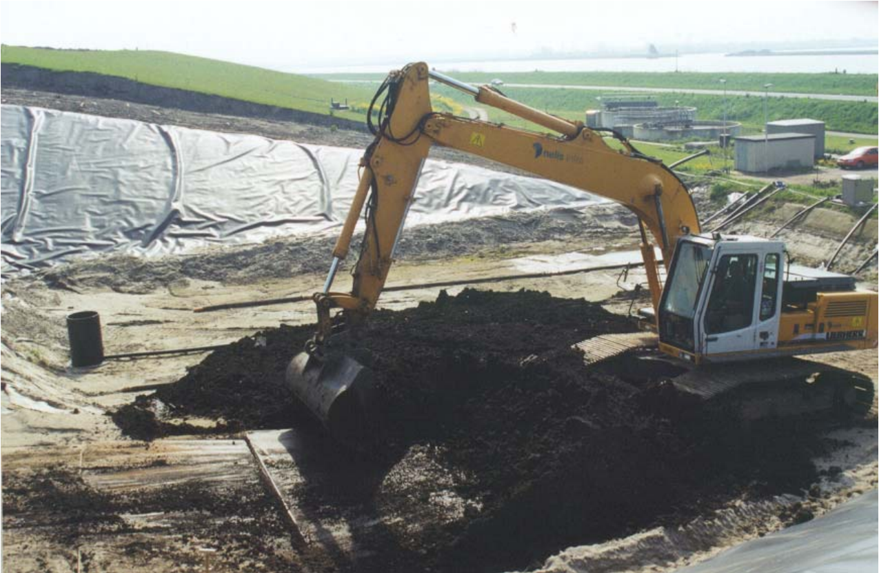
Figure 1. First batch of waste in the 12,000 m 3 pilot cell
